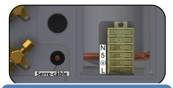
Step 2: Connect the connections housing and the outdoor unit through the cable tie with the 4G1.5 cord (not supplied) as shown in the wiring diagram (see section 3.5.4, p 21).
